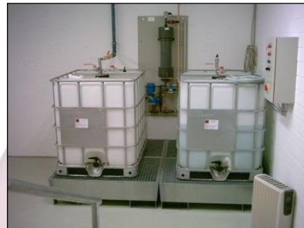
MA-3000 Central Formalin supply and disposal system with 600 litre containers for fresh and waste formalin
