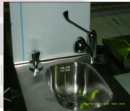
Sink with 25mm radius. Left : valve for operation of sprinkler system below work area
