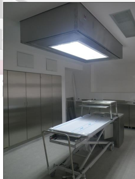
MA-2016 Air supply unit with integrated daylight source. Positioned within the ceiling
