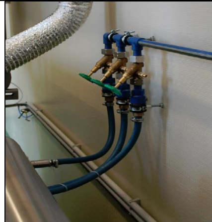
Example of the inlet at a maceration unit with 2 chambers (middle tap for supplying the shower)
