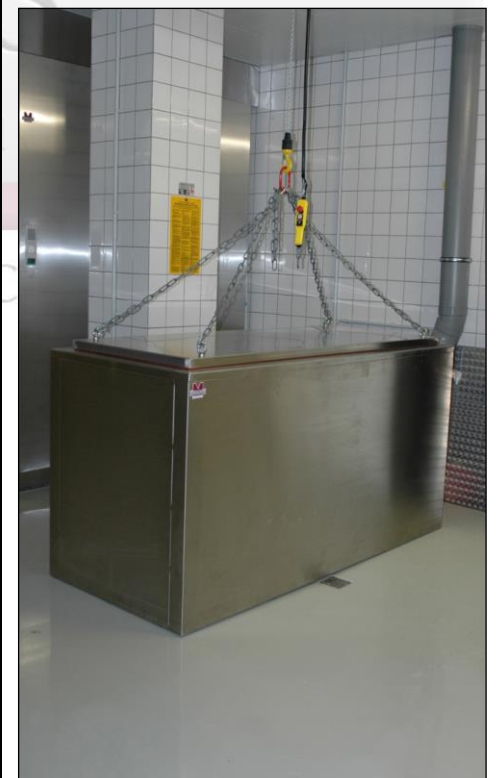
MA-1343.1 Preservation cuvette in a closed position. Extraction tube is lead to the ceiling
