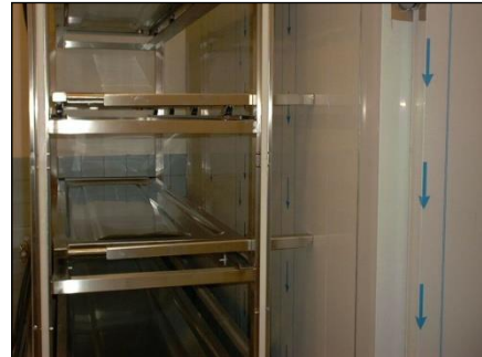
MA-1306 Body Tray Support with 3 levels inside a cold room
