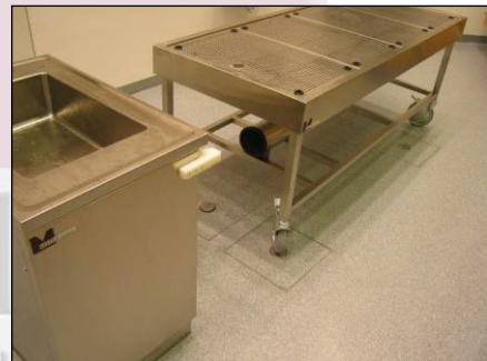
Air duct from dissecting table to docking station
