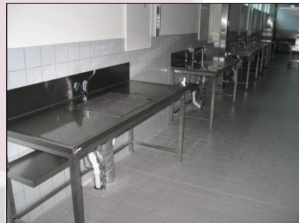
MA-0033 Tissue Grossing Tables with downdraft extraction for students
