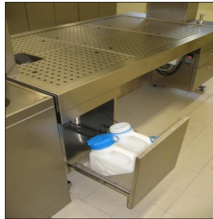
Integrated fresh formalin supply and used formalin drain system
